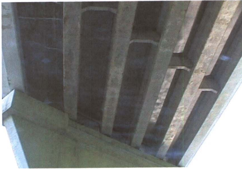
BOTTOM OF DECK
