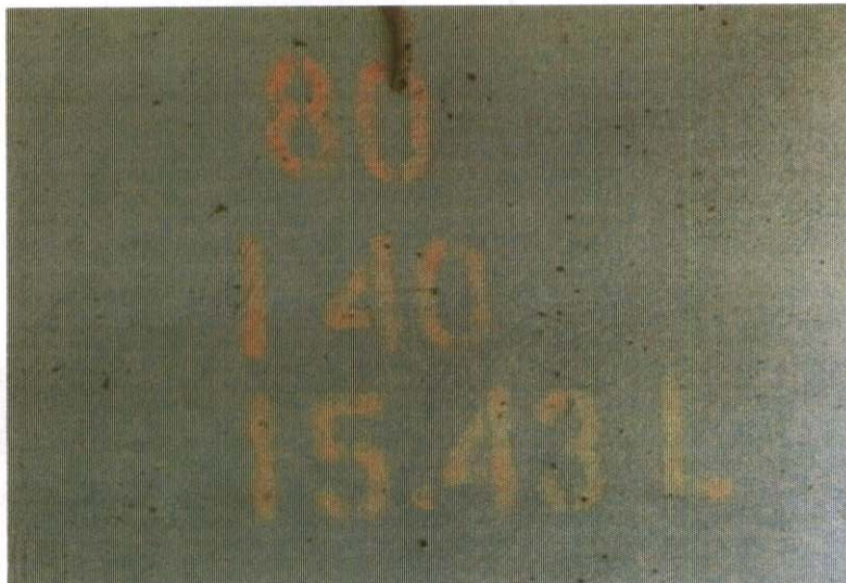
BRIDGE NO. AT ABUTMENT # 1
